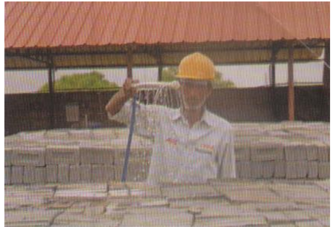
Treating ACC EcoBricks at the ACC Green Building Material Center
