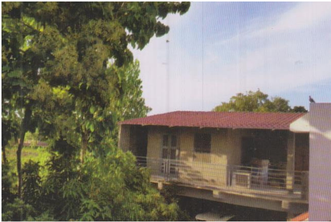
Completed house with material, expertise and manpower made available through ACC's GBMC
