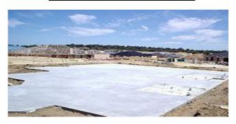
Shallow foundations are a type of foundation that transfers building load to the very near the surface, rather than to a subsurface layer. Shallow foundations typically have a depth to width ratio of less than 1.
